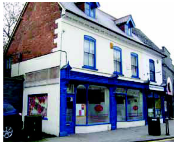
33, 35 and 37 Worcester Road
