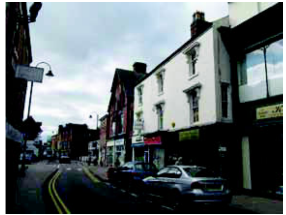
West side of Worcester Road
